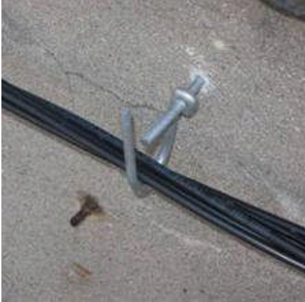
D Rings for Horizontal Cable Storage
