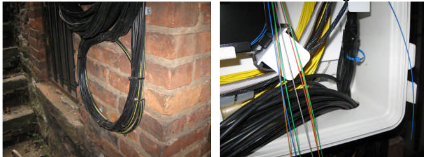
Maintenance coil storage and entering FDT.
